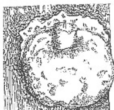
1. Candle in wet clay. The naked flame often caused gas to ignite and explode.
